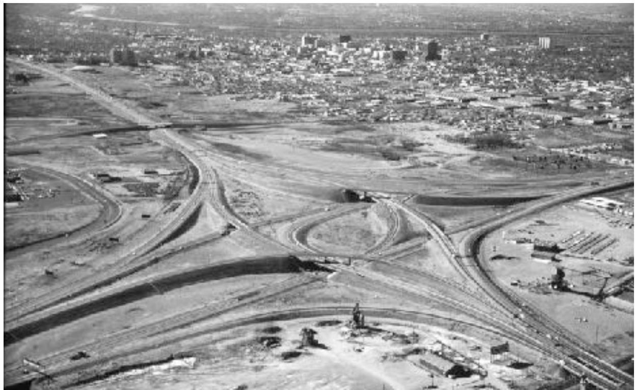
Photo of the construction of the "Big I" interchange, 1969, photo courtesy Albuquerque Museum PA1996.029.279
